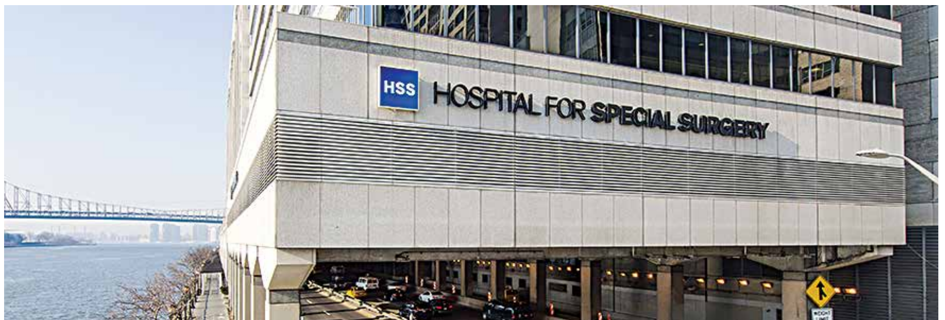
NEW VISTAS FOR JOINT EFFORTS: THIS NEW YORK NICHE HOSPITAL IS NOW HOME TO THE NEW STAVROS NIARCHOS FOUNDATION COMPLEX JOINT RECONSTRUCTION CENTER
