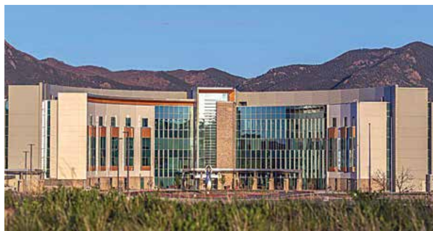
THE FUTURE IS NOW: THE COLO.-BASED CENTURA HOSPITAL GROUP IS NOW OPENING THIS HIGH-TECH BRAND-NEW HOSPITAL IN COLORADO SPRINGS, FEATURING "SMART" EVERYTHING
